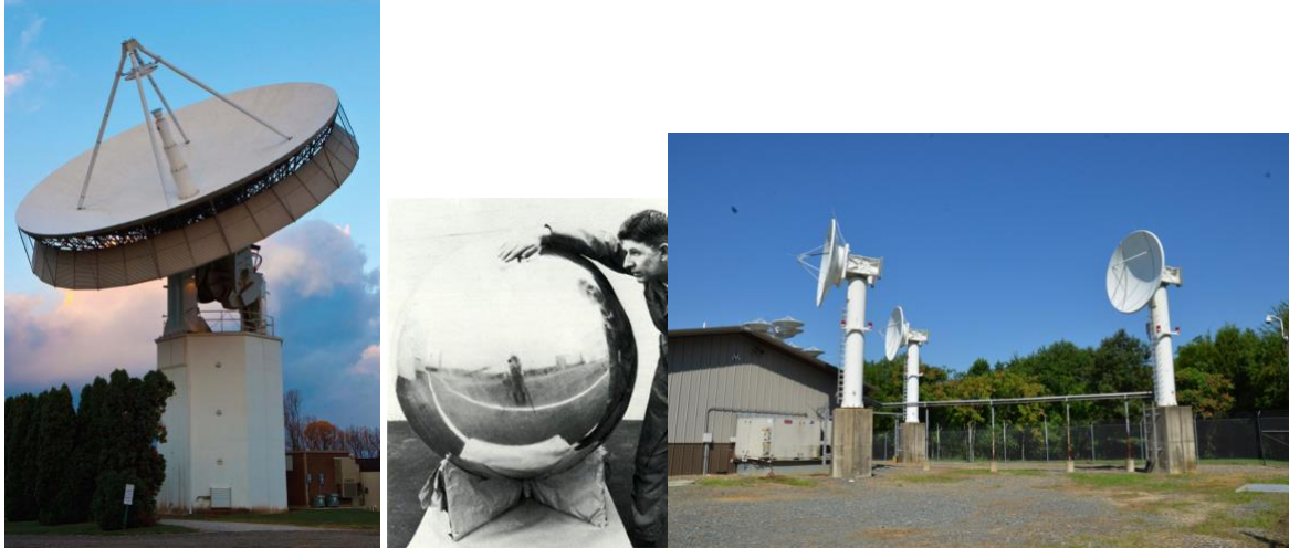
Figure 3 Left is the APL 18.3 Meter S-Band Ground Station Located in Laurel, MD Center: 1m Aluminum Sphere in low Earth Orbit Right: Three receive only antennas located on Stafford, VA
