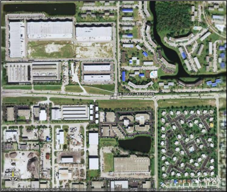
Figure 8. Aerial View, Site #4
