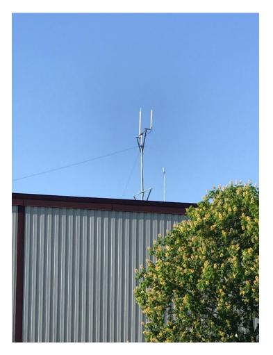
For this location, the building is 26 feet tall, the antenna structure is 18 feet, and the antenna itself will be 6 feet. In other words, the antenna will only extend 24 feet, or 7.3 meters, above the building. The height from the ground to the tip of the antenna will be 50 feet, or 15.2 meters.
