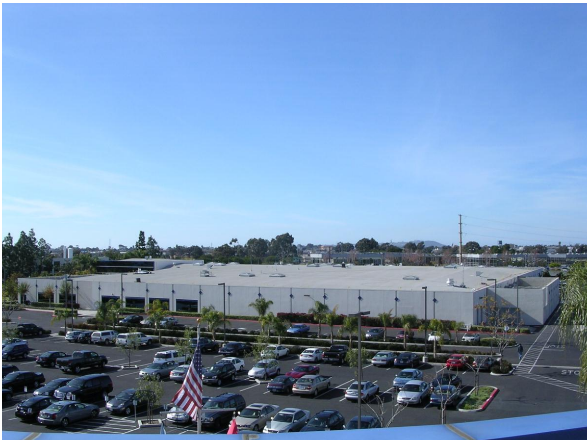
Figure 3. Rooftop, Building 8650, Expeditionary Warfare Center, San Diego, Ca.
