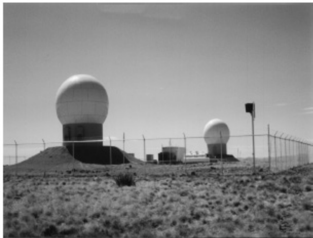
Figure 3-5 - The Radomes of a GES
