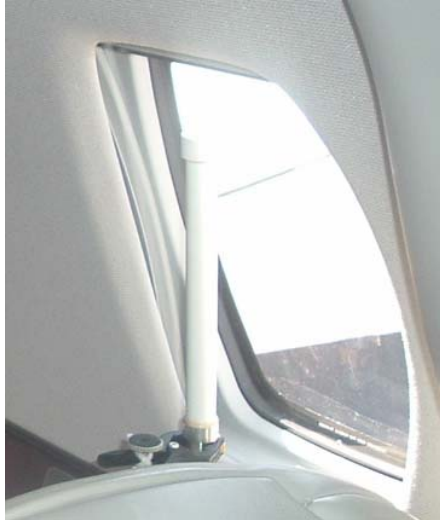
Figure 10. Typical inside PCS antenna location for ingress testing
