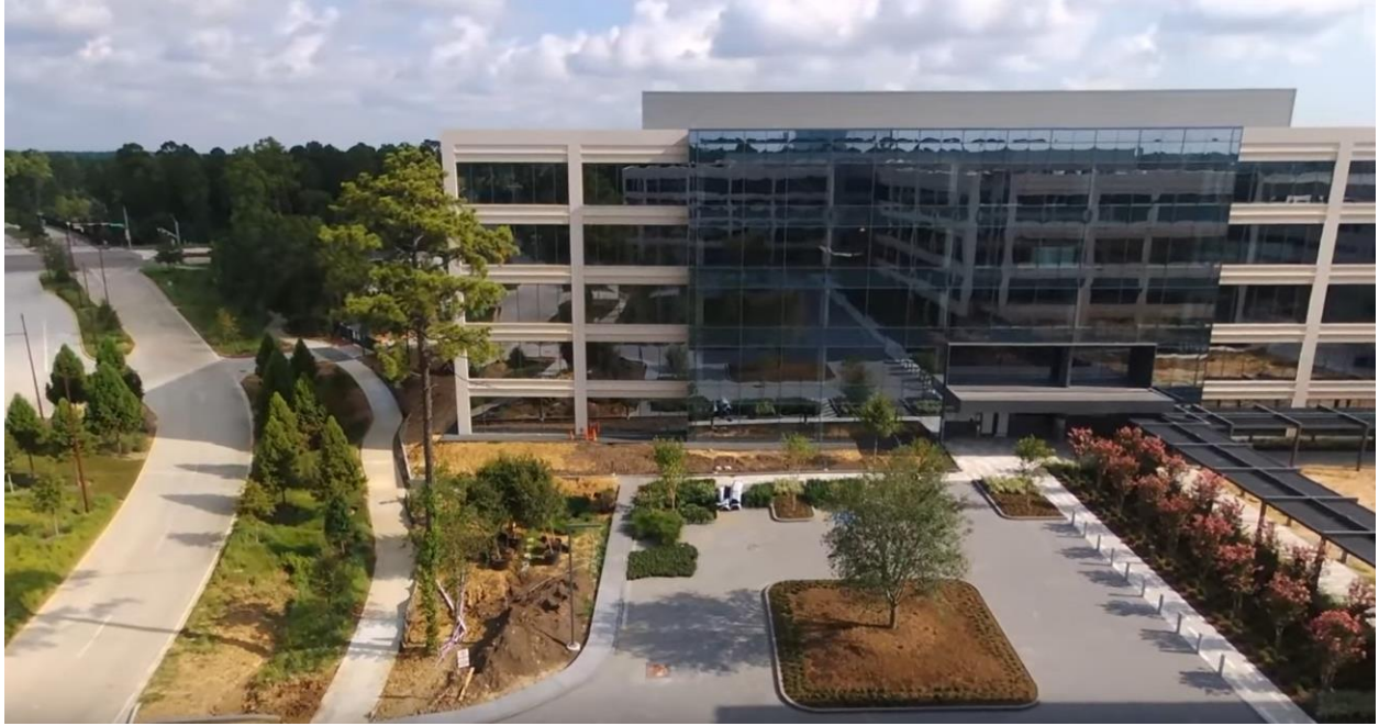
Figure 6 – View from outside of the HPI facility
