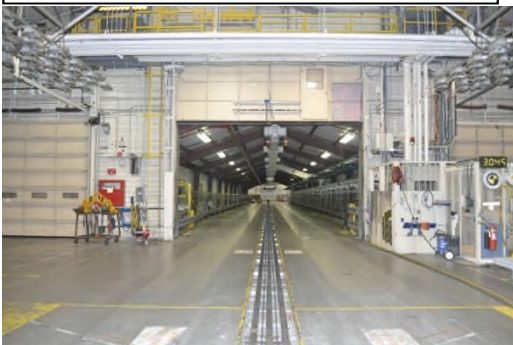
Figure 4 – Inside MPG Crash Test Building Facing South
