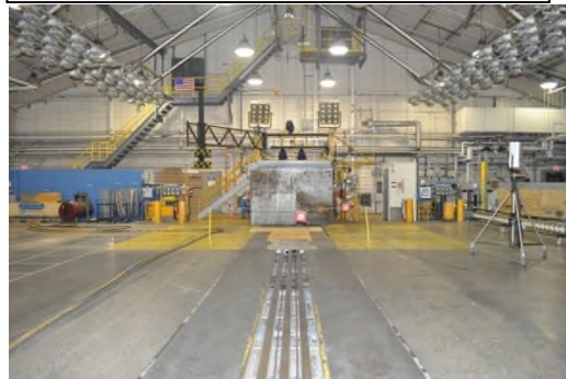
Figure 8 – Inside MPG Crash Test Building Facing North
