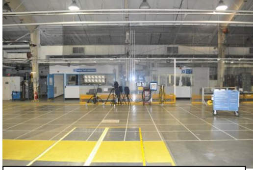
Figure 6 – Inside MPG Crash Test Building Facing West
