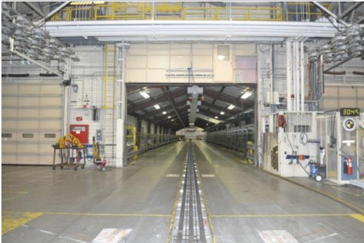
Figure 4 – Inside MPG Crash Test Building Facing South
