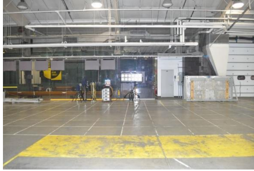
MPG Crash test building
