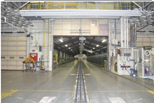
Figure 4 – Inside MPG Crash Test Building Facing South
