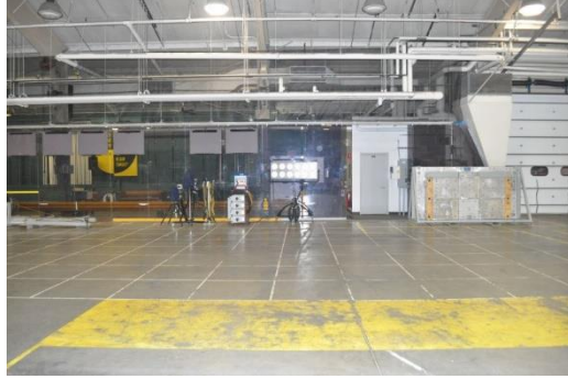
MPG Crash test building
