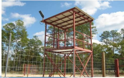
Tower: Detention Facility (1 each Corner)
