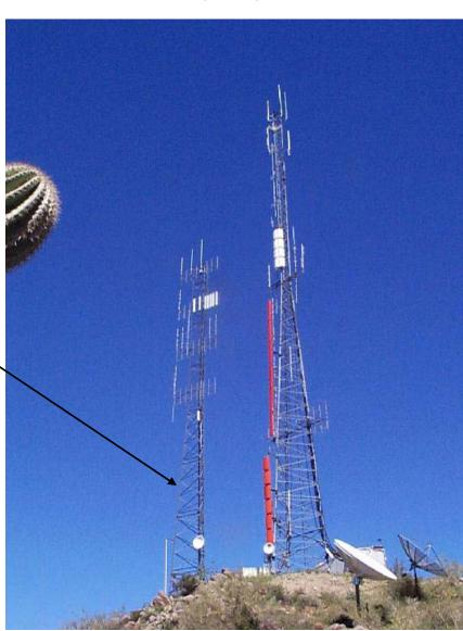
Antenna to be installed on East side of LMR tower at approx. 40' (12.2 m)
