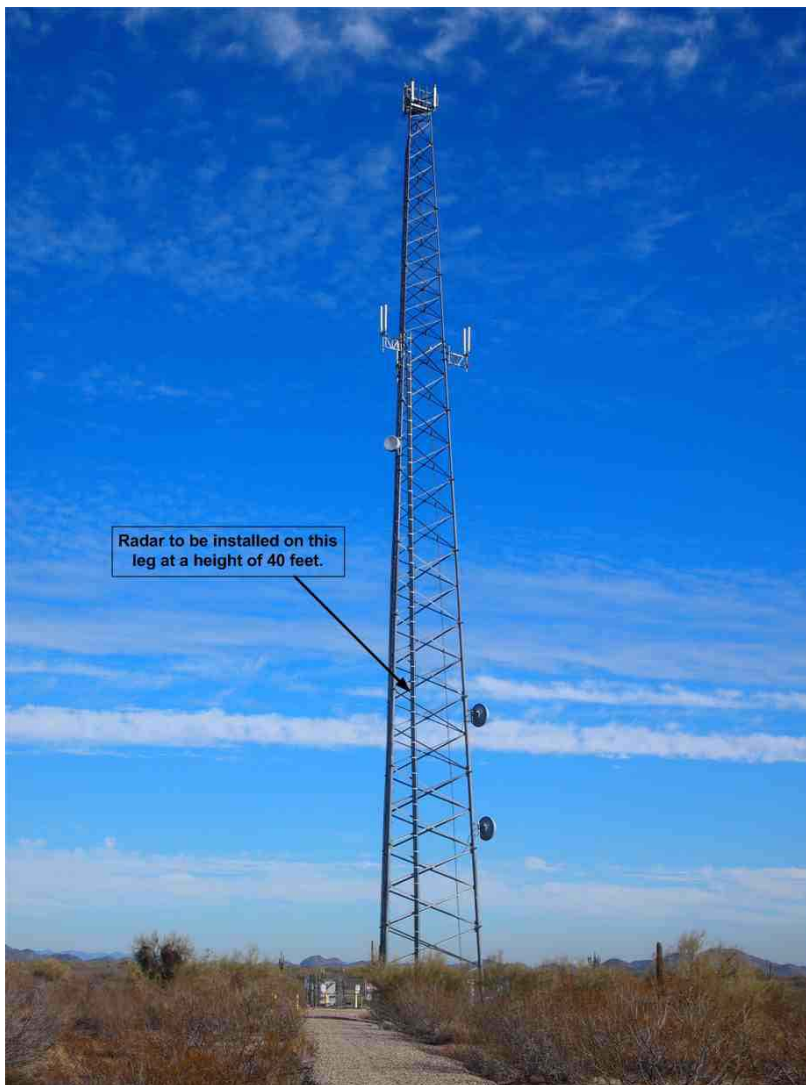
Figure 1 - Wittman Tower (looking east)
