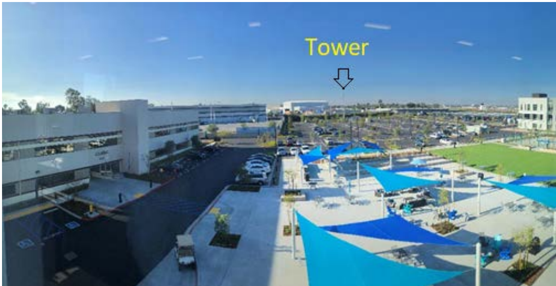
Figure 2. Panoramic view from East to South to West of company campus.
