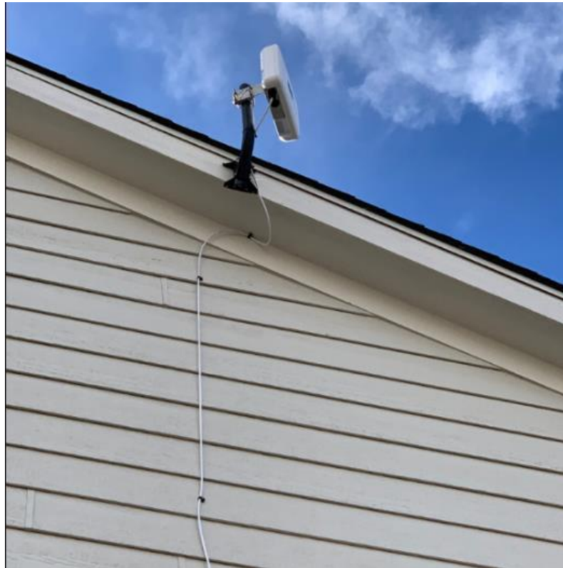
Example device installed at a customer premise with wiring connecting to the PoE
