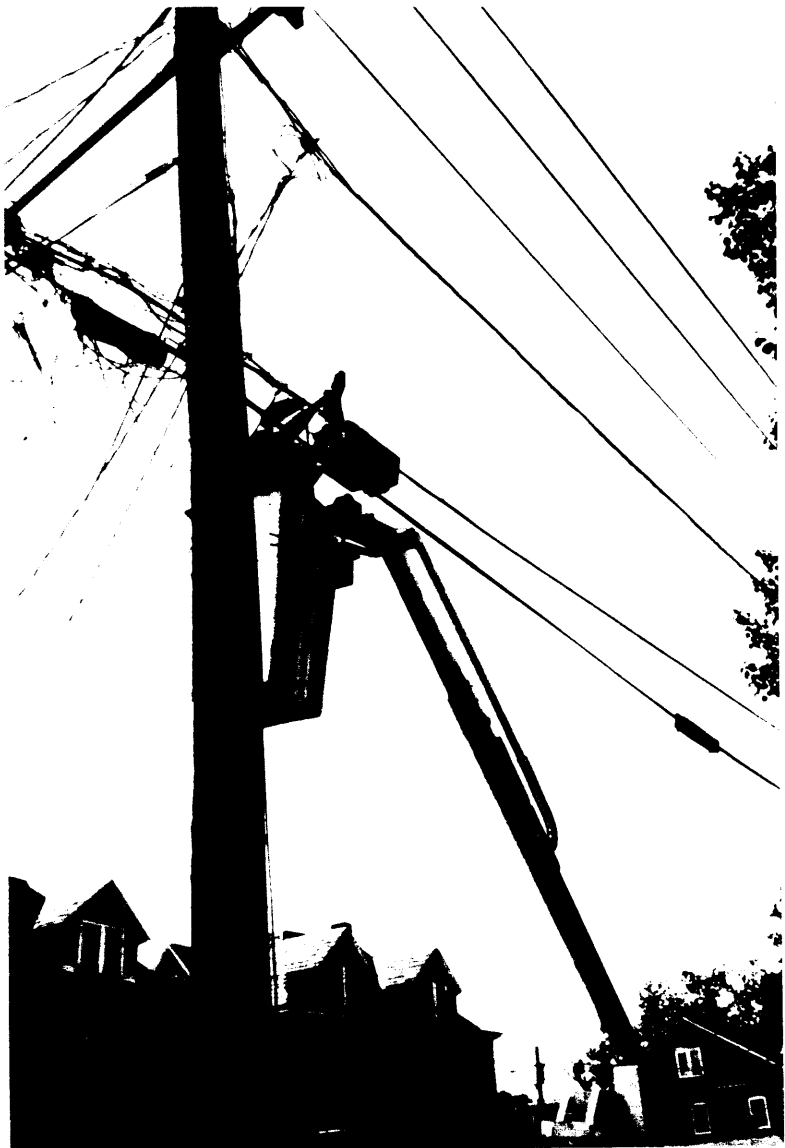
FIGURE 12 - INSTALLATION OF OUTDOOR ANTENNA PORT CD
