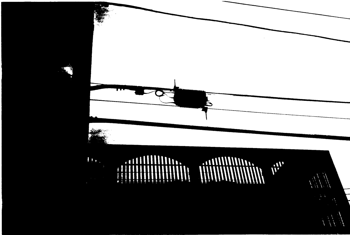
FIGURE 11 - INSTALLATION OF OUTDOOR ANTENNA PORT AB
